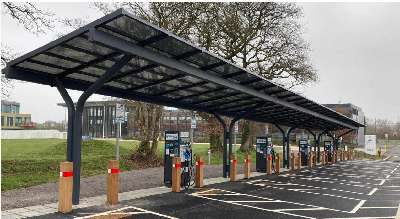
Figure 27: Best practice example - Bristol and Bath Science Park: As part of the Revive network, an EV charging hub was installed at Bristol and Bath Science Park, led by South Gloucestershire. This hosts 12 EV charging bays, including 5 rapid chargers and 1 fast charger. The charging bays are covered by a transparent solar glass canopy which both protects users of the hub from the elements and generates electricity. Whilst this is not a residential charging hub, lessons can be learned on how to design a hub effectively .
